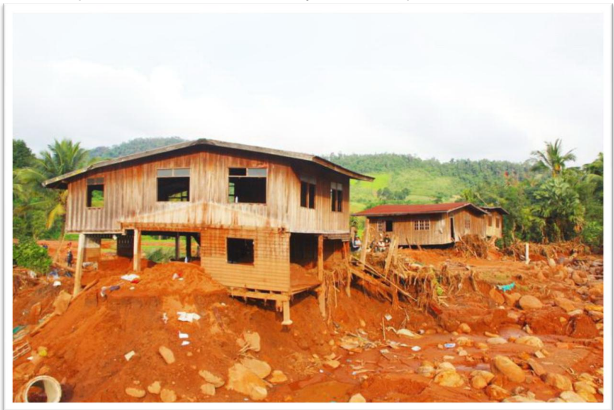
Photo 4. Cooperative Member's House washed by Flood (13 th Sept. 2011)
